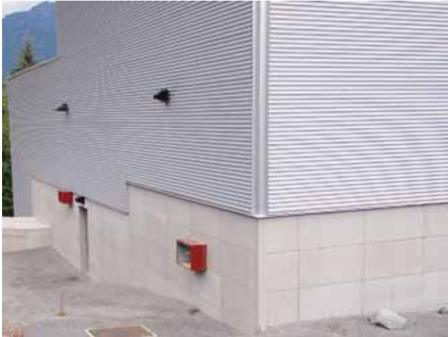
Refrigeration Plant, Whistler B.C.
